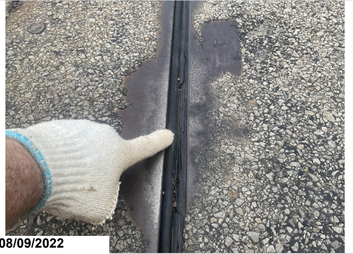
Abutment 1 expansion joint-Cracking with rips
