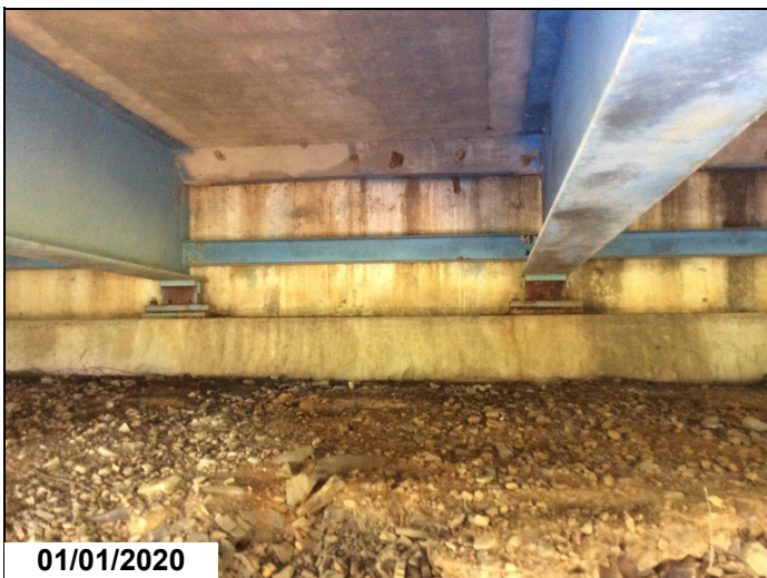
Corrosion on the bearings.
