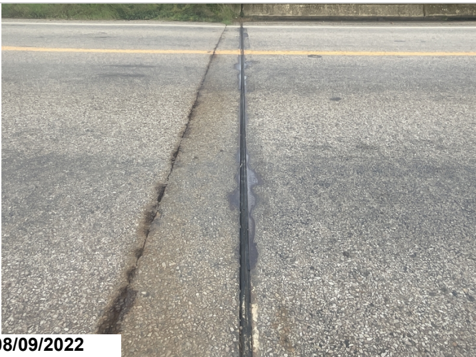
Abutment 1 expansion joint
