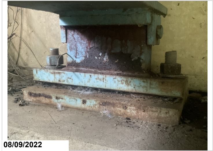
Abutment 2, bearing 1-Corrosion
