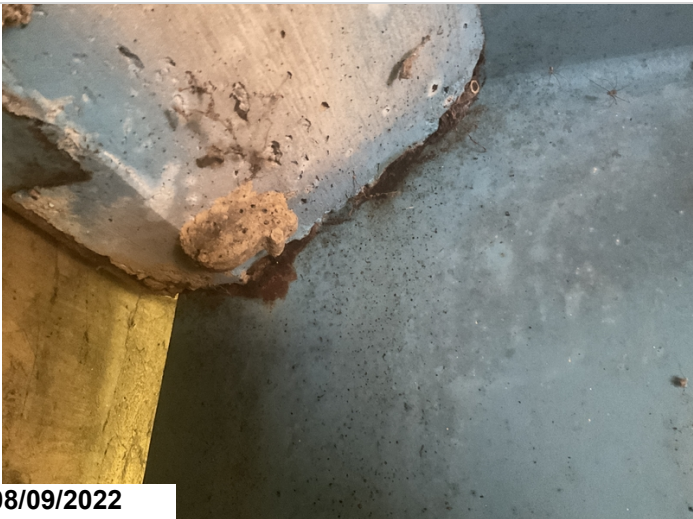
Abutment 2, beam 4-Corrosion at expansion dam
