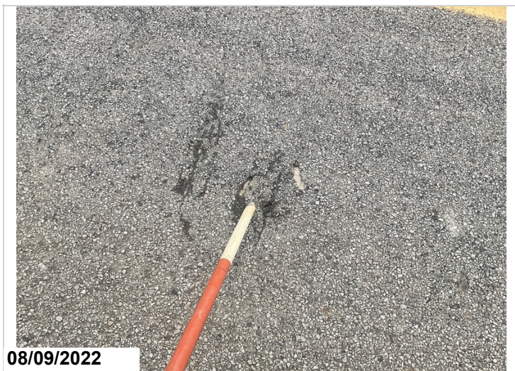
Chip and seal wearing surface has areas of scrape marks and gouges in the left lane.
