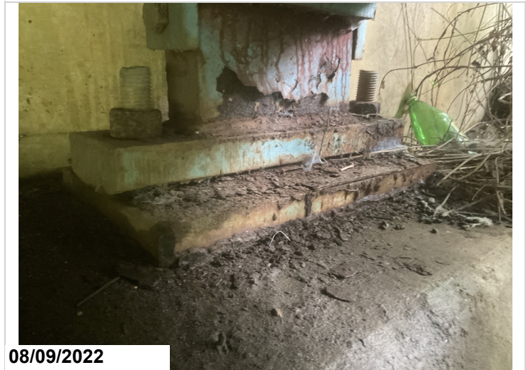
Abutment 2, bearing 4-Corrosion with pack rust between rocker and masonry plate.
