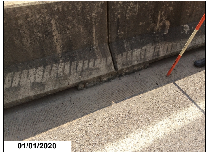
The base of the concrete parapets have areas of shallow spalling with exposed reinforcing steel.
