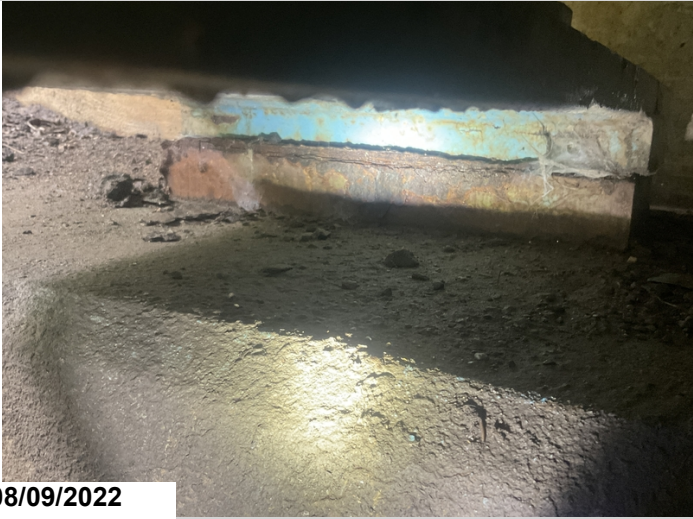
Abutment 1, bearing 4-Corrosion
