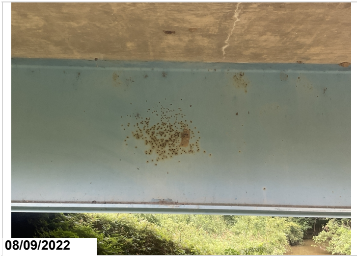
Beam 4 exterior side-Apparent impact from shotgun
