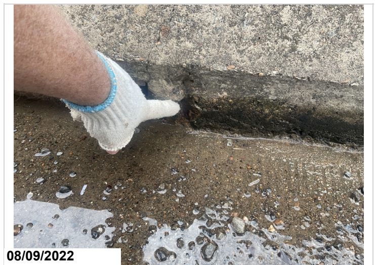
Right parapet-Shallow spall with exposed reinforcing steel
