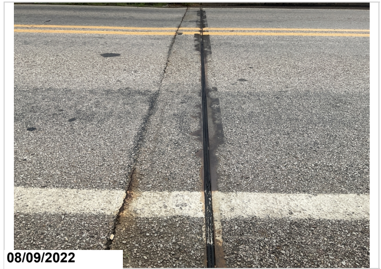
Abutment 2 expansion joint
