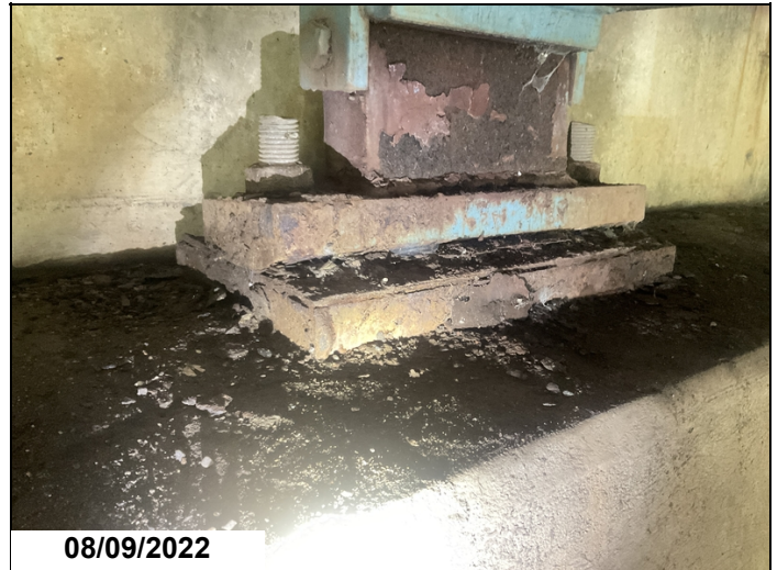
Abutment # 2, bearing # 3-Corrosion with pack rust between rocker and masonry plate.
