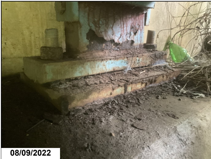
Abutment # 2, bearing # 4-Corrosion with pack rust between rocker and masonry plate.
