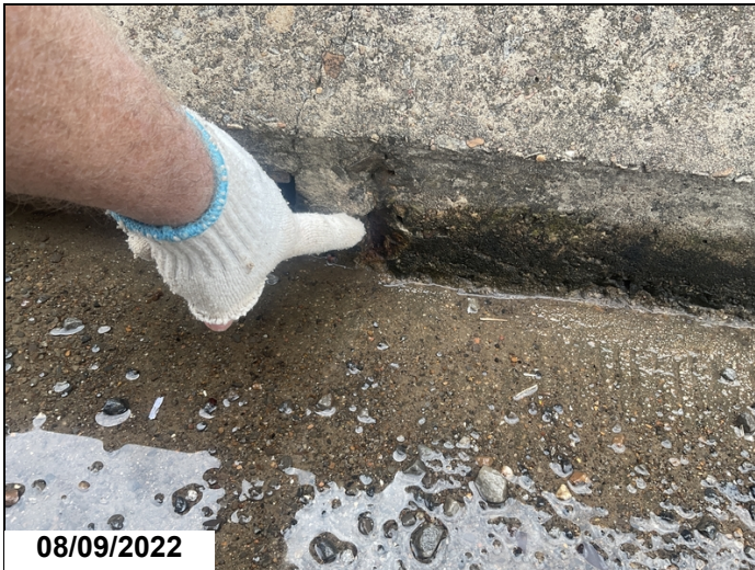
Right parapet-Shallow spall with exposed reinforcing steel.
